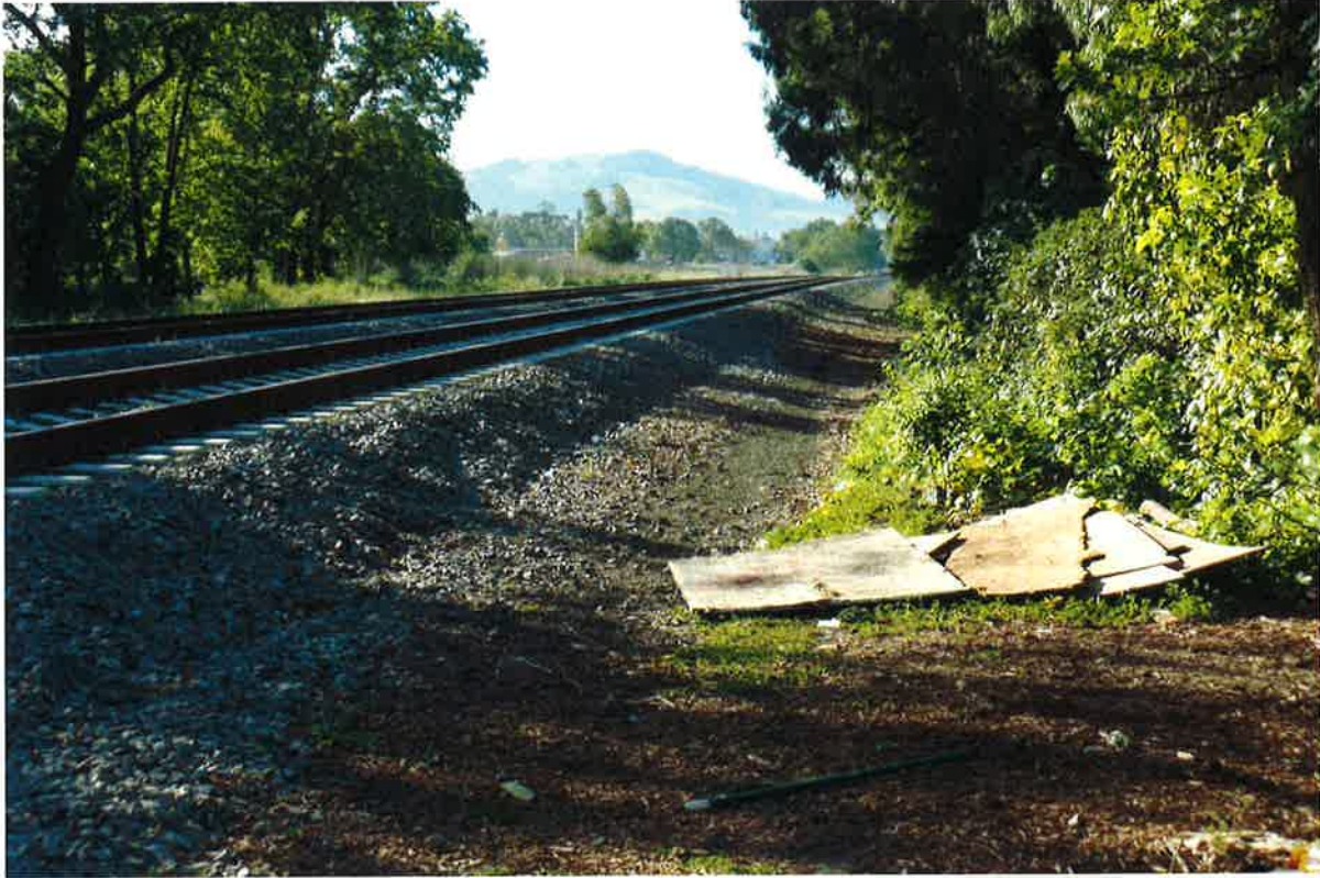
Standing 17 feet from centerline of rail on the west side of the rail looking south
