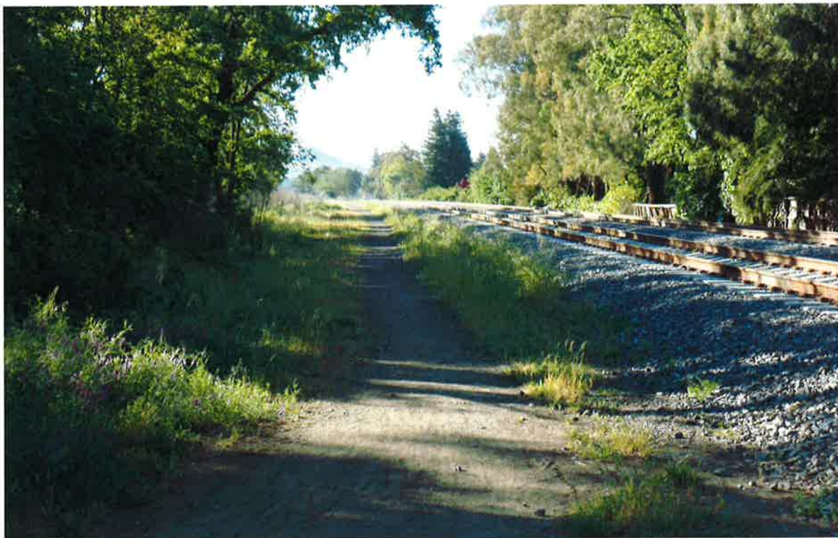
Standing 17 feet from centerline of rail on the east side of the rail looking south.
