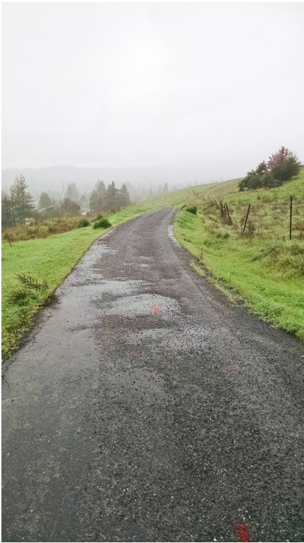
A: Existing access road looking west.
