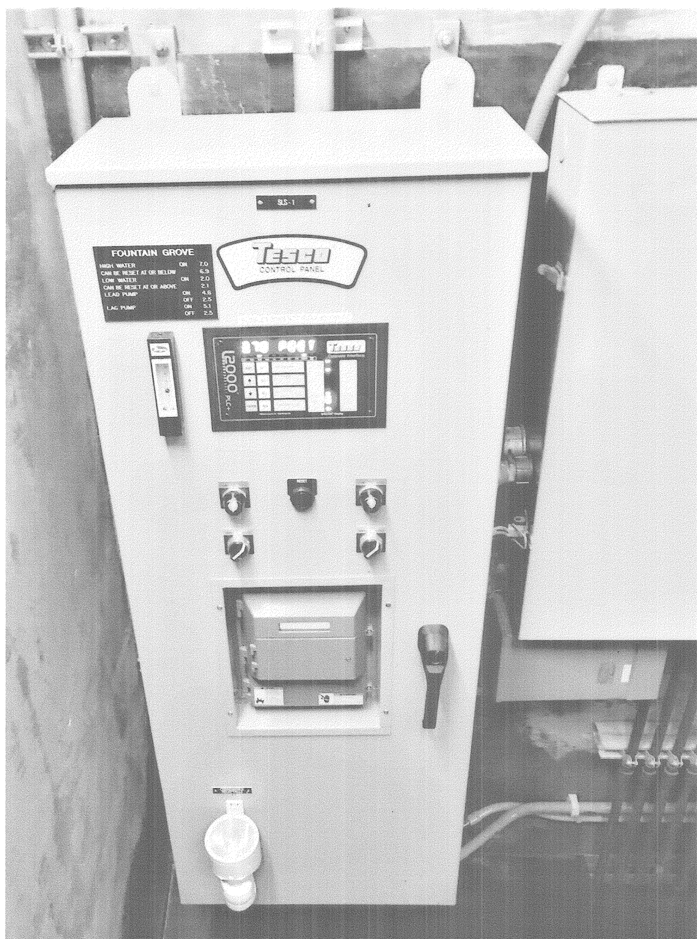
SEWER LIFT STATION SLS 1 SCALE: NTS
