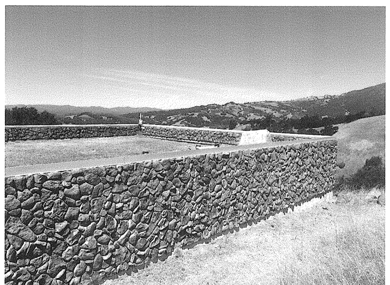
10 - NORTHEAST EXTERIOR BUILDING FACE
