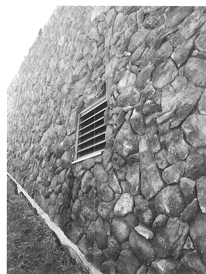
3 - LOUVER TO REPLACE
